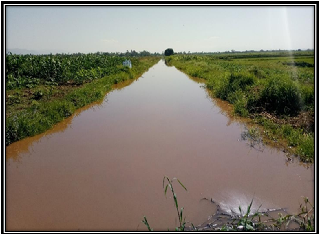
Figure 4.2: Well-maintained irrigation canal without aquatic weeds.
