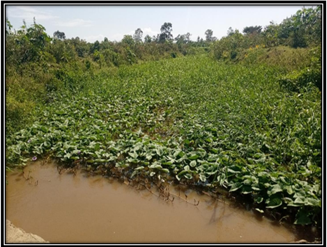
Figure 4.1: Poorly maintained irrigation canal with aquatic weeds.
