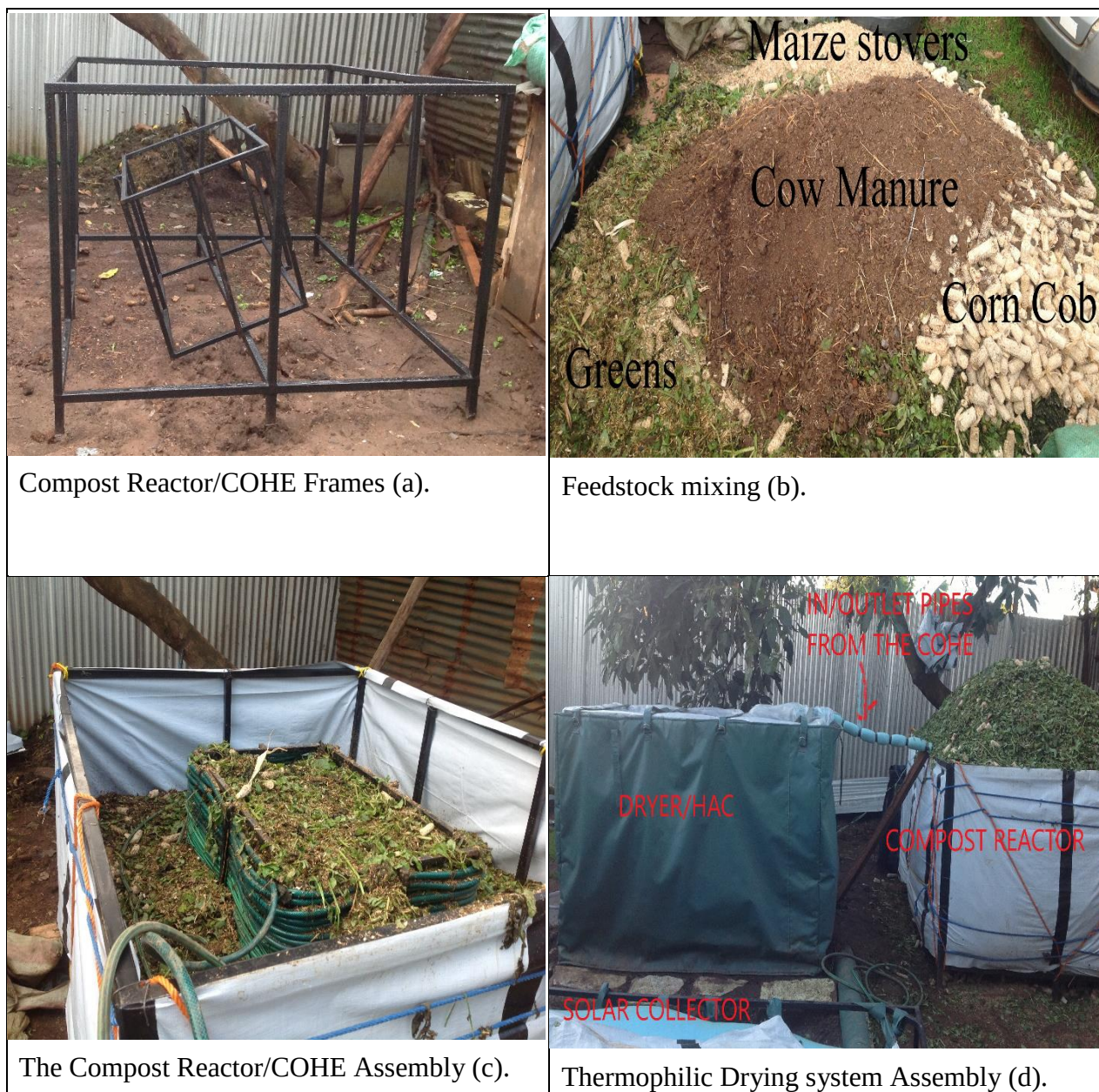
Figure 3.2:Pictorial view of Compost Reactor/Compost Heat Exchanger Site development.
