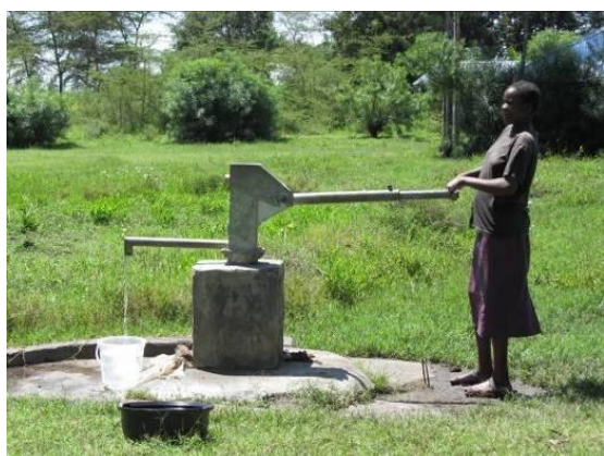
a: protected hand pumped well
