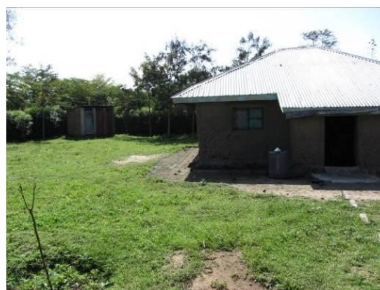
b: roof rainwater harvesting
