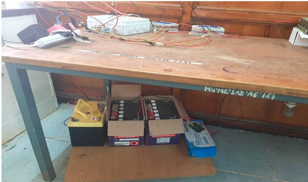
Figure 3.10: Data logger and batteries (storage)
