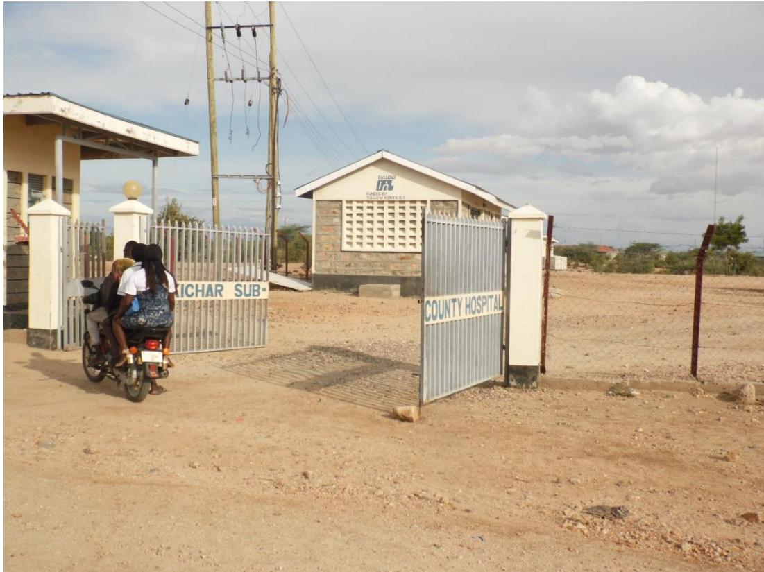
Plate 8: Section of Lokichar Sub-County Hospital Built by Tulow Oil Co.
