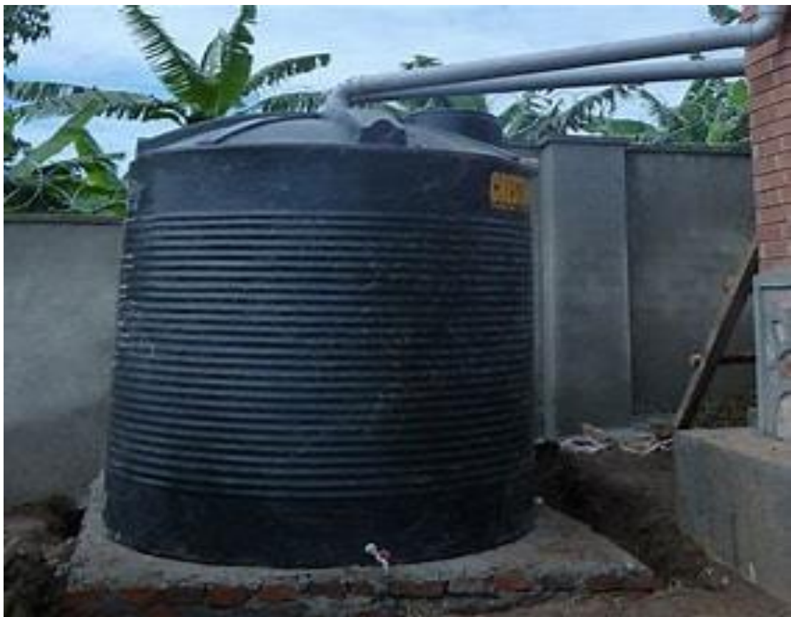
Plate 4.3: Showing rain water harvesting using a plastic tank and gutters, in Makindye division
