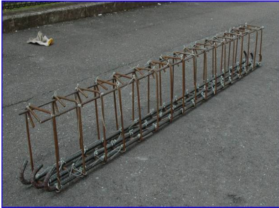
(a) Large beam stirrup-rebar's cage
