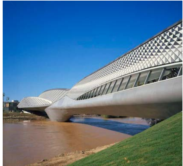
(a) Concrete bridge decks and piers
