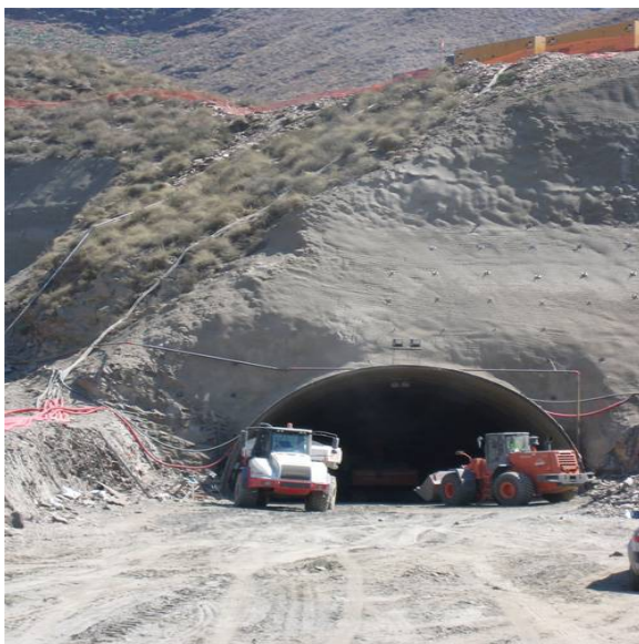
(c) Tunnel linings and slope stabilization
