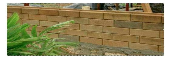
**Figure 4.3** A wall built using interlocking stabilized soil blocks The respondents were however neutral on fire resistance of soil (mean, 3.97), low energy input in processing ISSB(mean, 3.69) and that production of ISSB is labour intensive therefore creates employment(mean, 3.98). The respondents were also neutral to the idea that ISSB production and construction uses cheap local labour (mean, 3.89).
