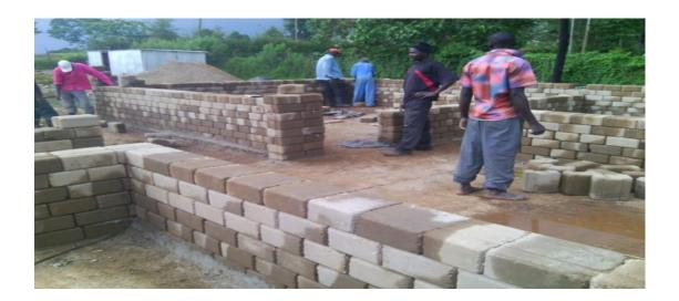
**Figure 4.2.** A house under construction using ISSB The blocks in figure 4.2 are joined to form neat joints that do not require further rendering
