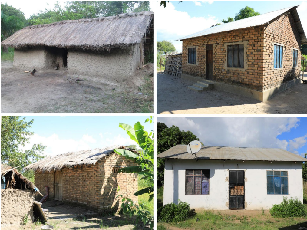
Fig. 2 Pictorial representation of typical local house types in the study area. Top left: a house with grass thatch roofing with mud walls. Top right: a house with corrugated iron roof and brick walls not plastered on the outside, and sometime also not plastered on the inside. Bottom left: grass thatch roof with brick walls not plastered on the outside, and sometime also not plastered on the inside. Bottom right: a house with iron sheet roofing and plastered brick walls. A variety of window and door designs and covers are also illustrated
