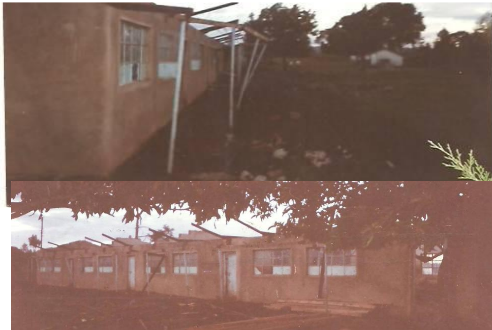
Figure 4.1: A school block destroyed by wind at a primary school in Nandi Central District
