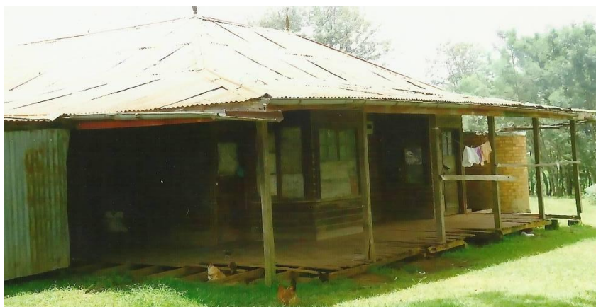
Figure 4.6: Old white- Settler Houses used as teachers' quarters
