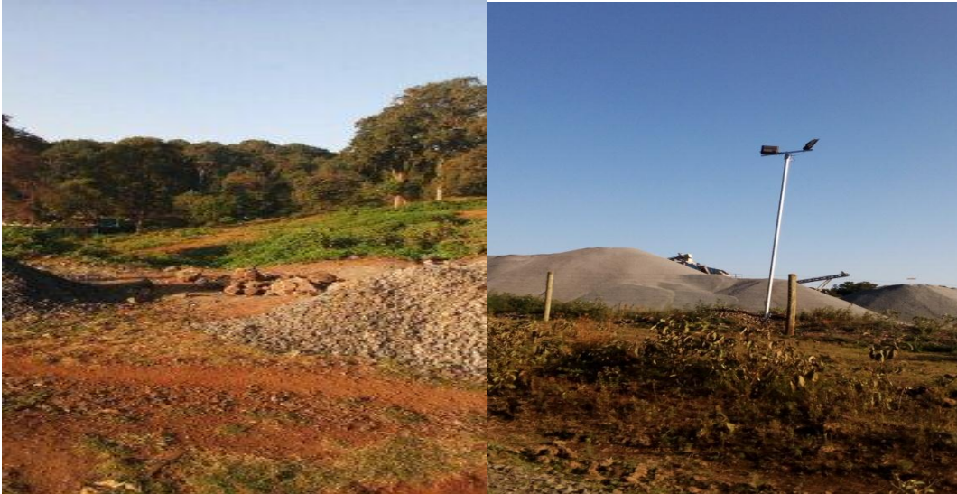
Plate 2: Stone blasting near Meru technical college (left) and Murram deposit (right) along Naari foot path
