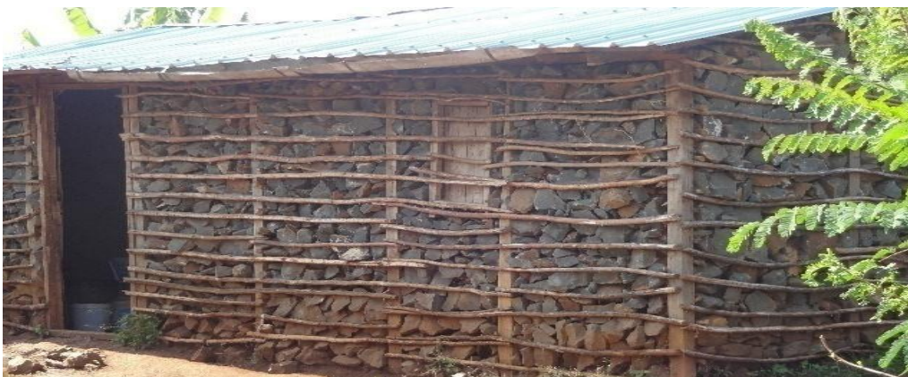
Plate 4.10: Reinforcing of house walls using stones in Amani
