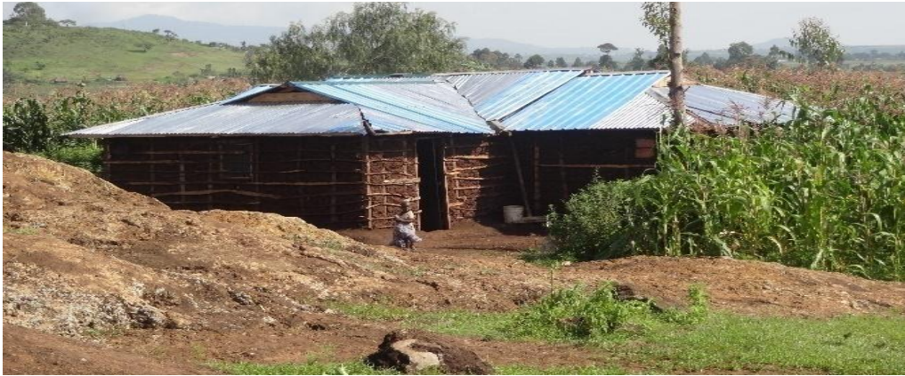
Plate 4.9: Reconstruction of houses with bigger rooms and improved quality
