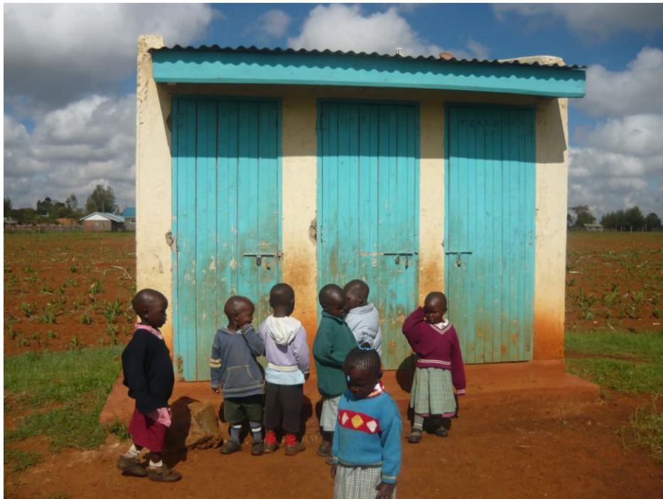
Fig. 5.4.2.4 A Toilet constructed through CSG
