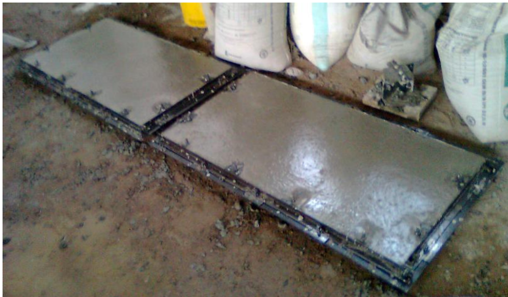
Figure 3.28: Freshly placed slab panel elements
