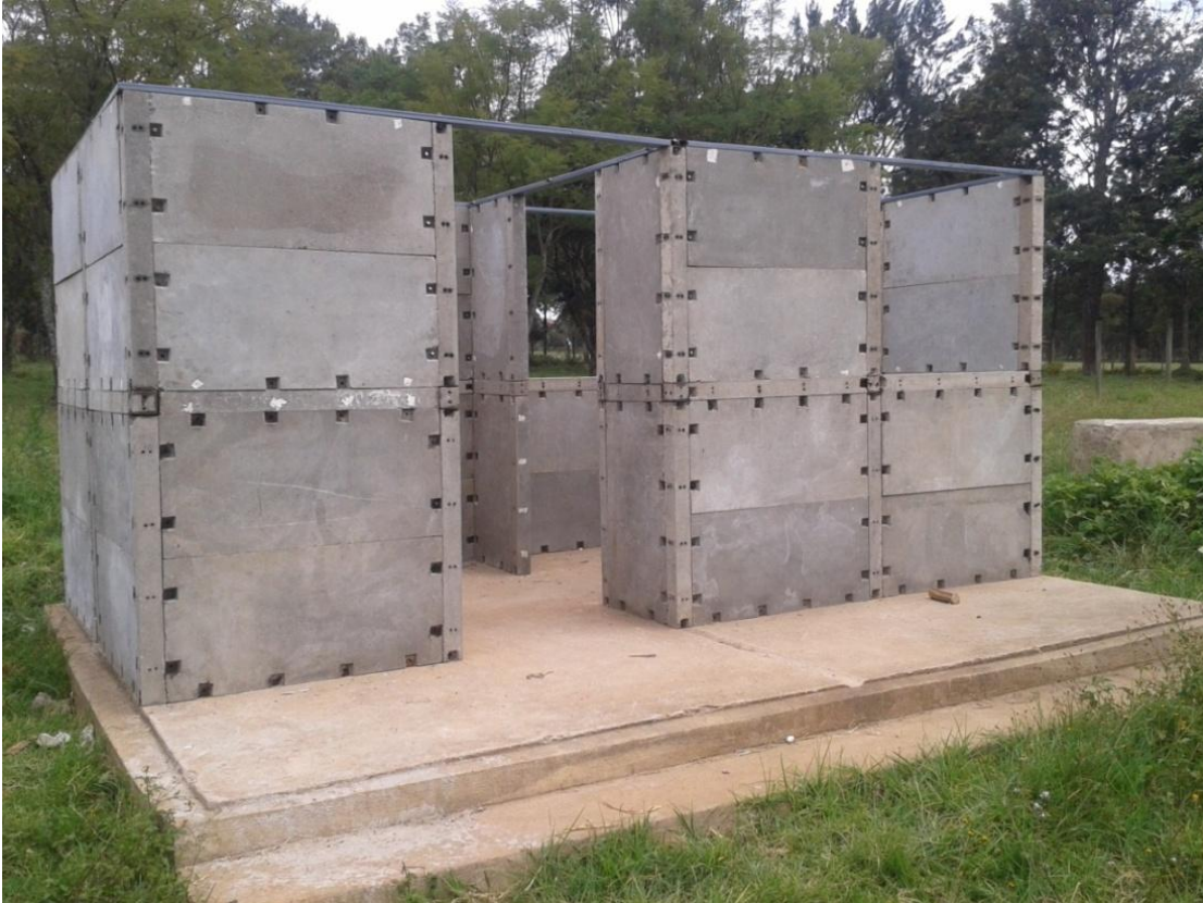
Figure 4.14: Construction stage 2 completed with openings for doors and windows
