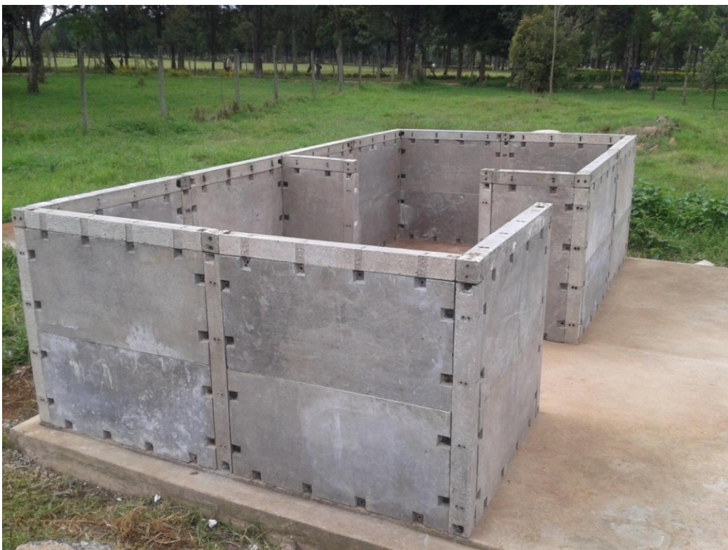
Figure 4.10: Construction stage 1 in progress, single panel assembled from the inside
