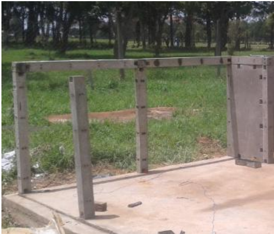
Figure 4.727: Picture of the development of the framework of beams and columns
