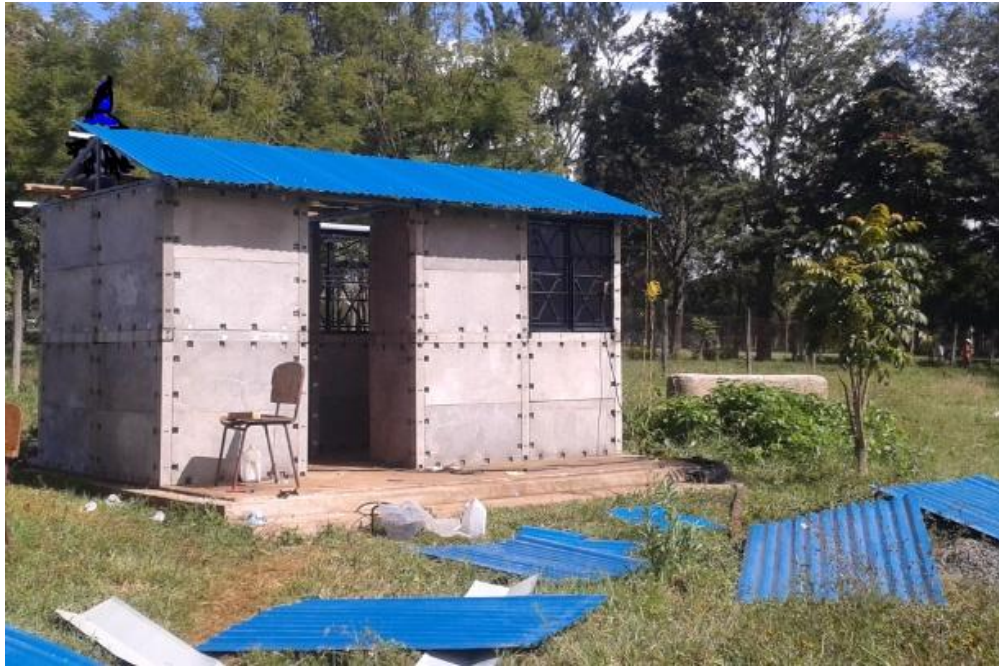
Figure 4.1733: Roofing work in progress
