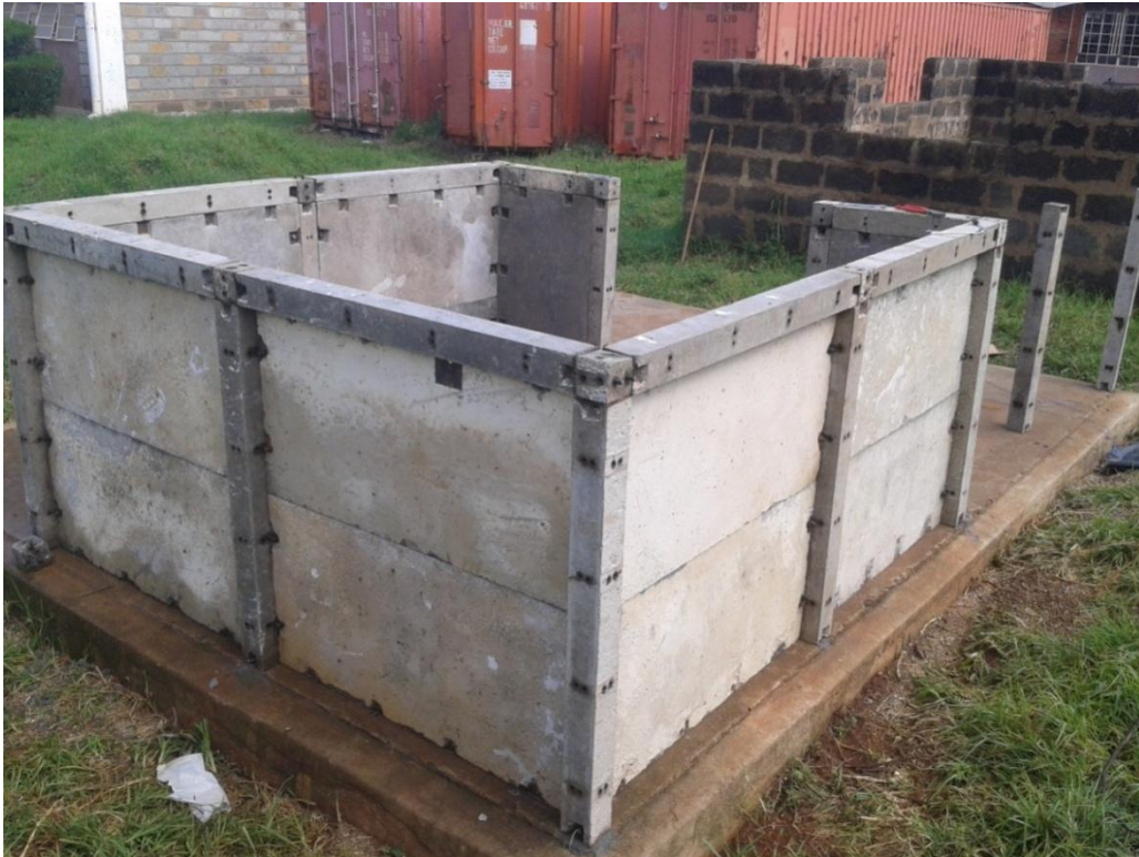
Figure 4.10: Construction stage 1 in progress, single panel assembled from the inside
