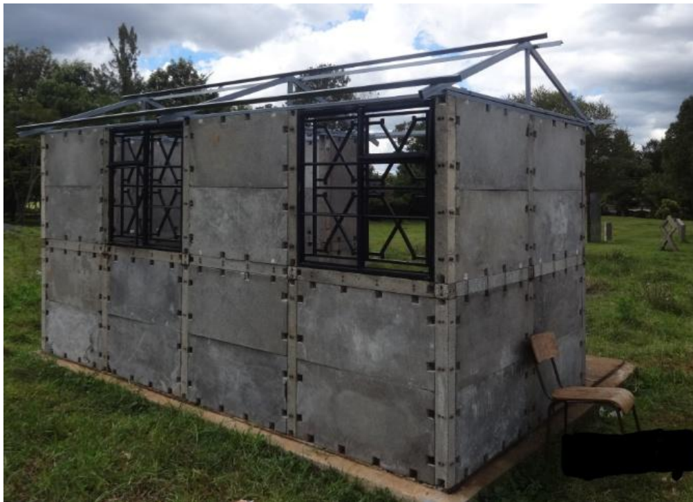
Figure 4.1632: Roof trusses mounted and window frames fitted
