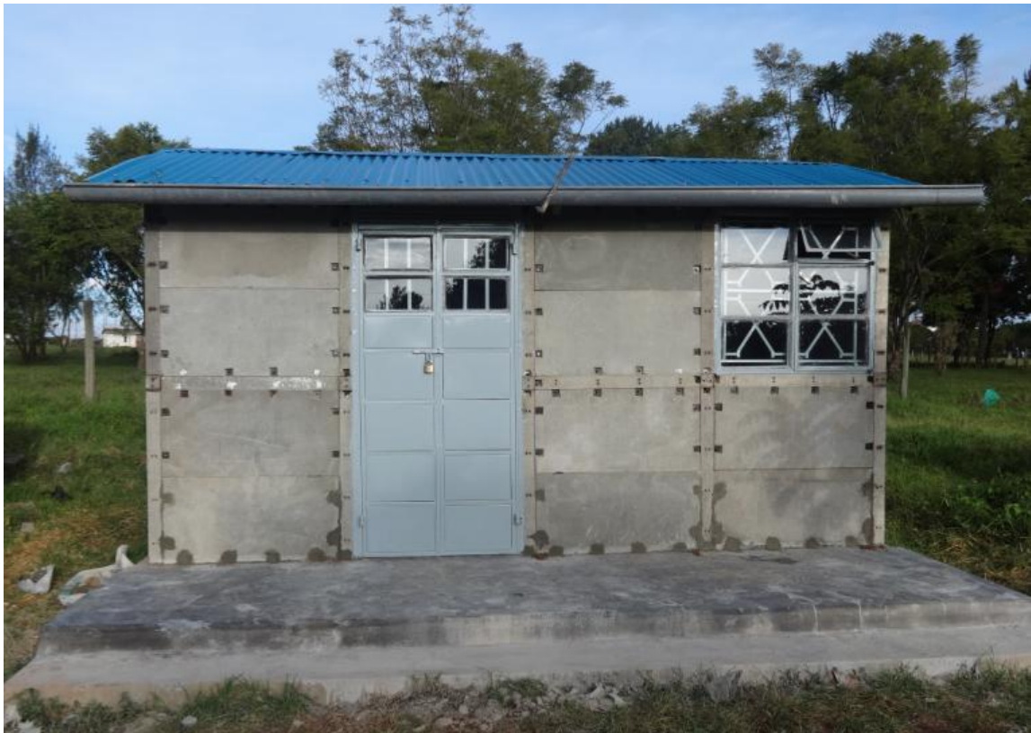
Figure 4.1935: Completed Pilot House
