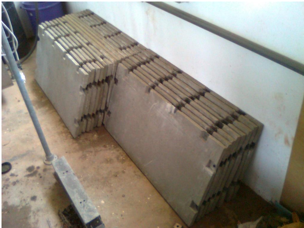
Figure 3.2921: Slab panels transported and stacked
