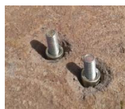
Figure 4.424: Anchor bolts dropped into bolt-hole for fixing column, and column already fixed
