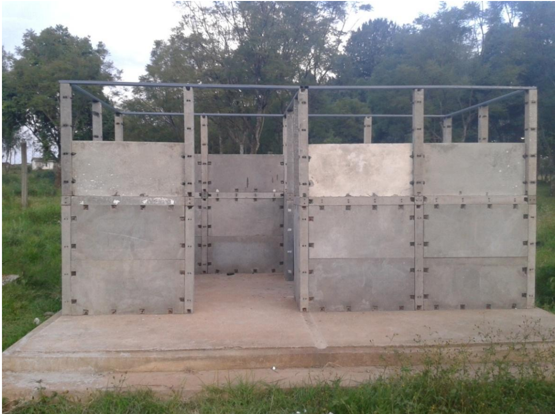
Figure 4.1331: Construction stage 2 in progress
