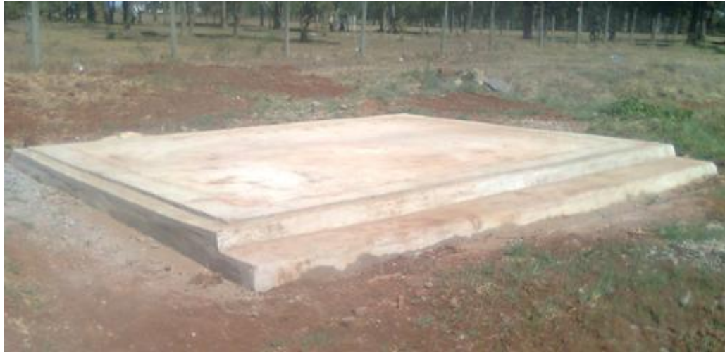
Figure 4.122: Image of the finished floor
