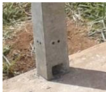
Figure 4.424: Anchor bolts dropped into bolt-hole for fixing column, and column already fixed
