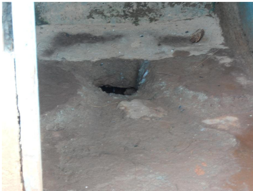
Plate 11: A chipped latrine floor that results in increased aperture size
