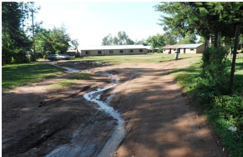
Plate 9: Expansive compound at Ichina primary school without a fence and designated gate
