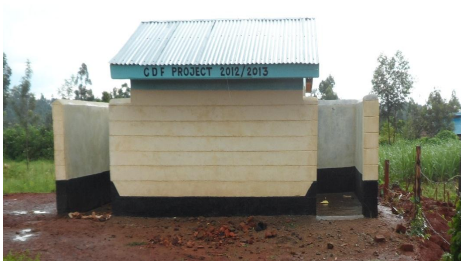
Plate 14: Newly constructed sanitary block at Nyayo Tea Zone primary school (was not in use at the time of study)
