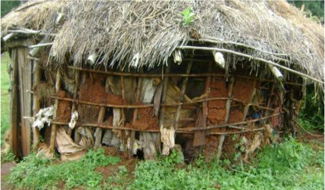
Condition of the wall.
