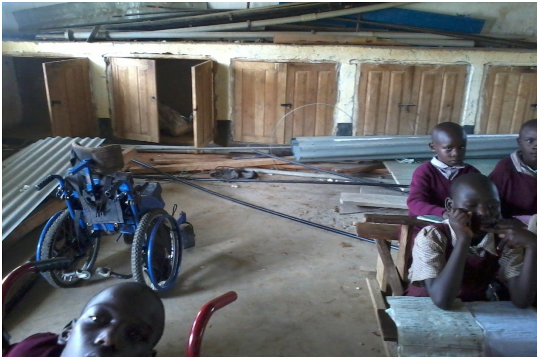
Plate 4.8: Presence of inaccessible Store Boxes within a classroom
