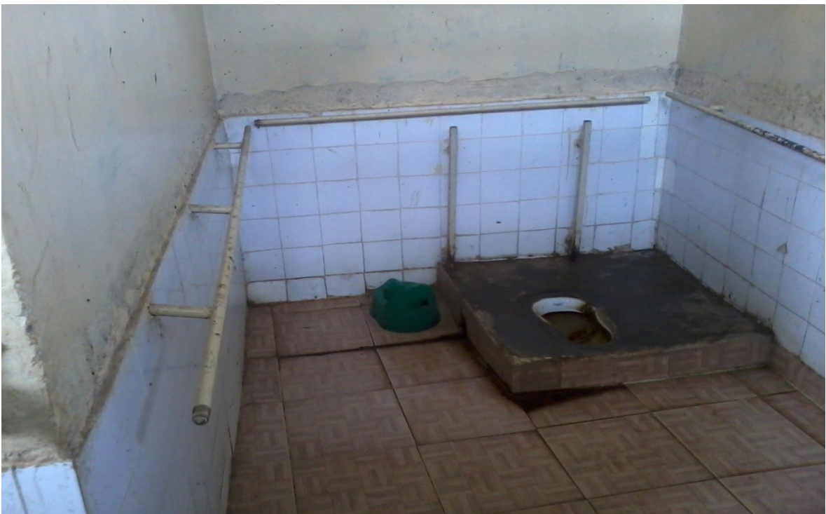
Plate 4.15: Presence of Adapted toilets with Holding Rails Used by Pupils with Physical Challenges
