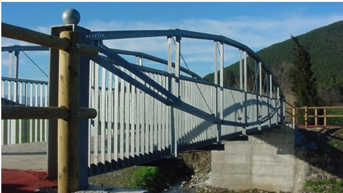
Figure 1.16: Bardena river footbridge in Italy 10
