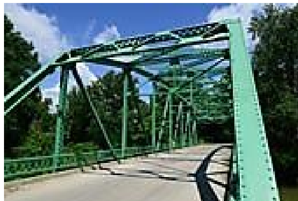
Figure 1.11: Howe Truss Bridge 5 .
