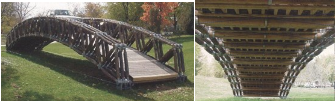
Figure 1.8: Light pre-stressed segmented arch bridge.
