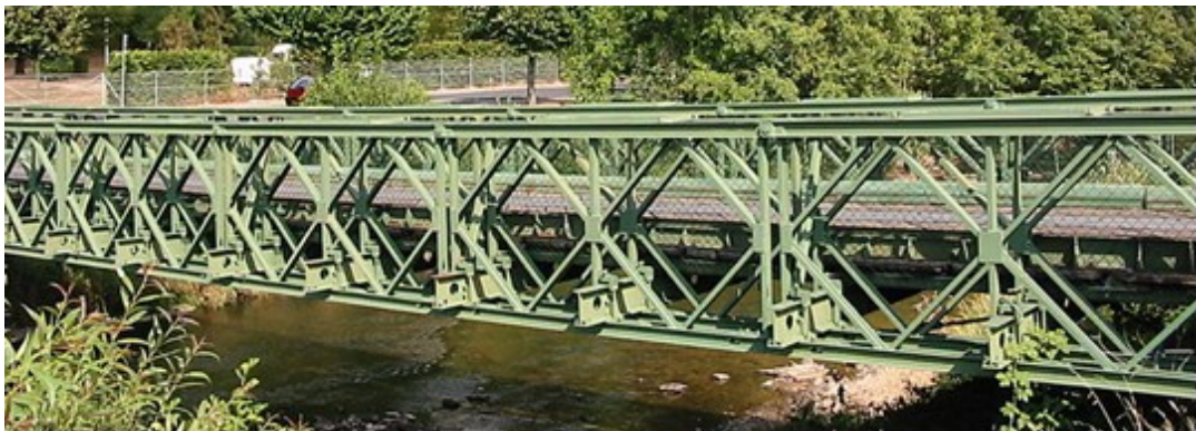
Figure 1.13: Bailey bridge over the Meurthe River in France 7
