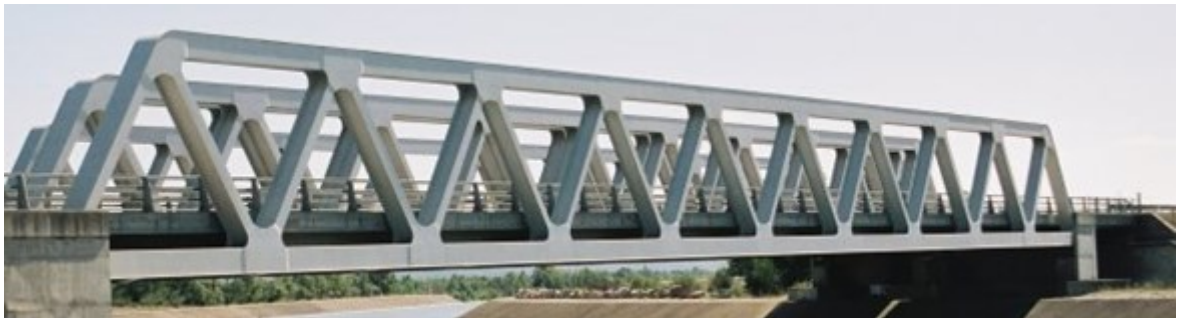
Figure 1.9: Sainte-Tulle Bridge in France 3 (Warren Truss).
