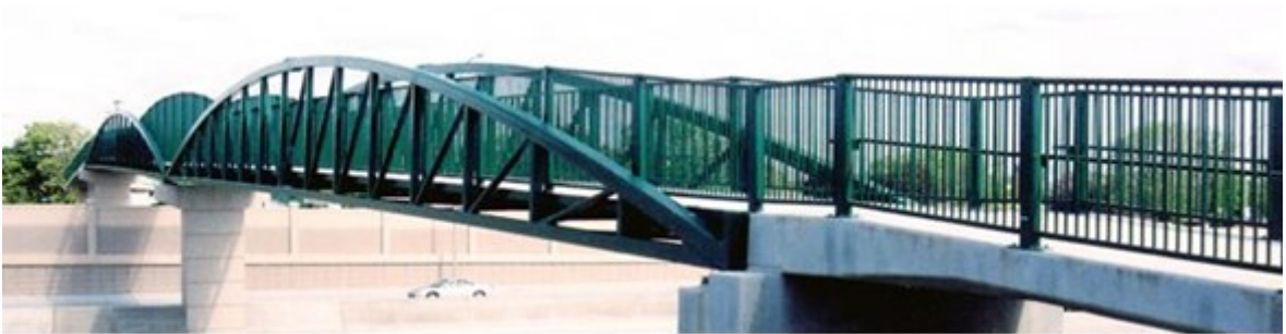
Figure 1.14: Bowstring truss bridge in Rochester Minnesota 8
