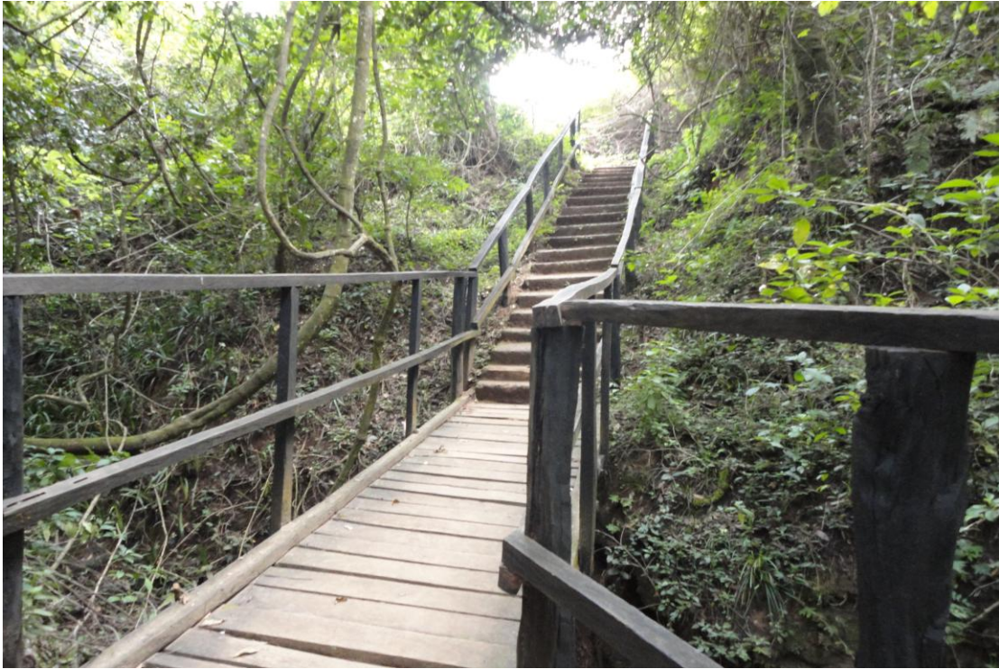
Plate 4. 7: A Bridge and foot path in the Nature trail
