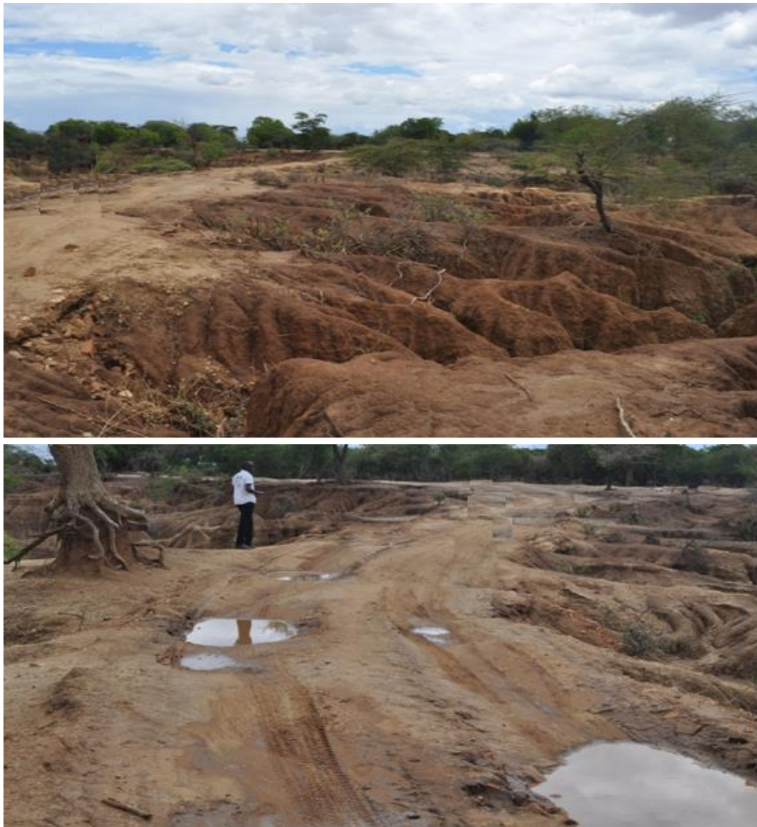
Plate 4.7: The State of the Roads in Serewo Area
