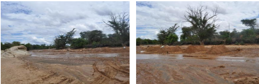
Plate: 4.16 Photo of Widened River Banks
