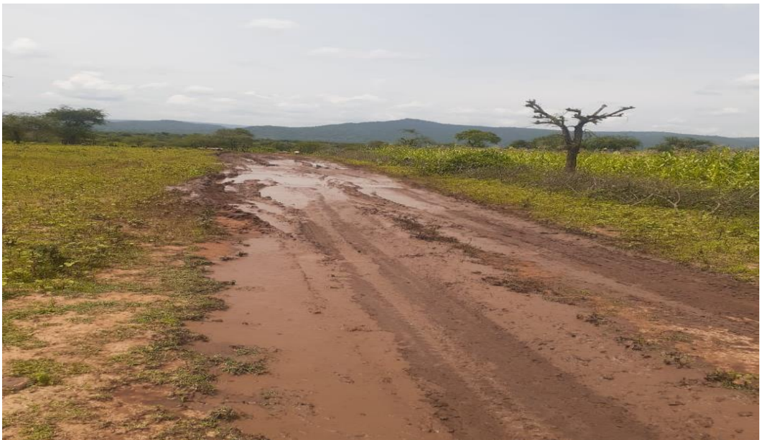
Plate 4.9: State of the Road in Kanyarkwat
