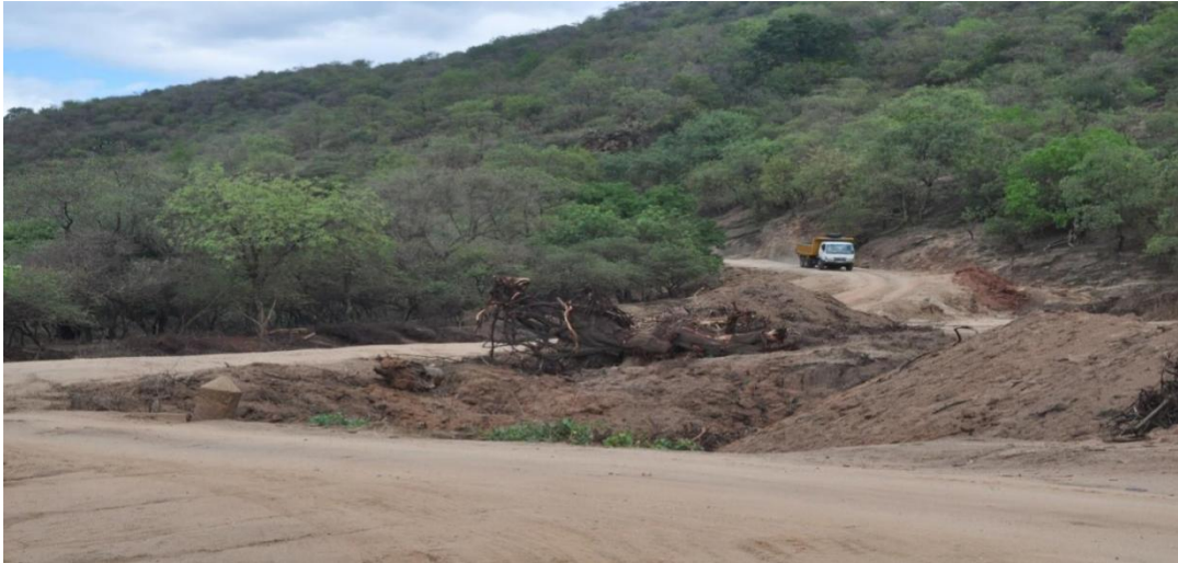
Plate 4.8: State of the road in Mtembur
