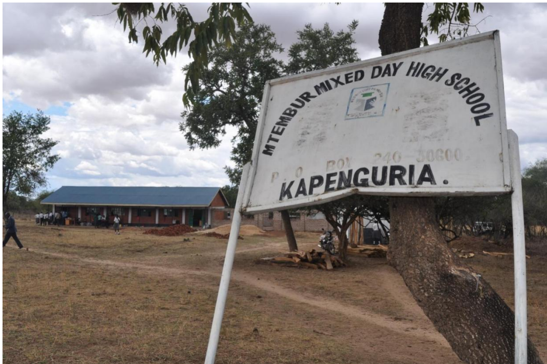
Plate 4.10: A class room funded by Mtembur CBO
