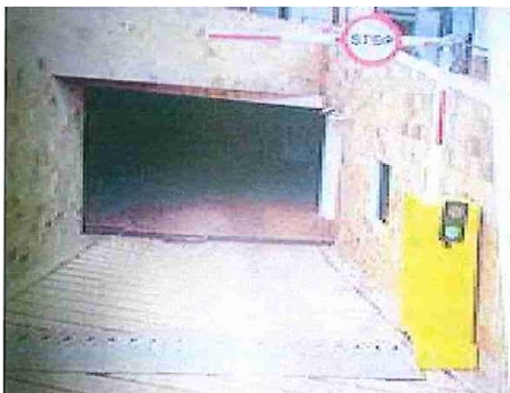
Fig 7: Automated gate barrier
