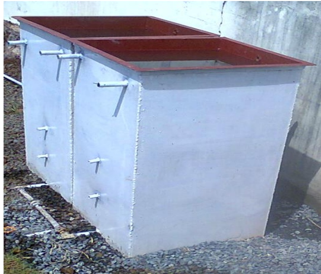
Figure 3.4 Two Dynamic Gravel Filters (DyGFs)
