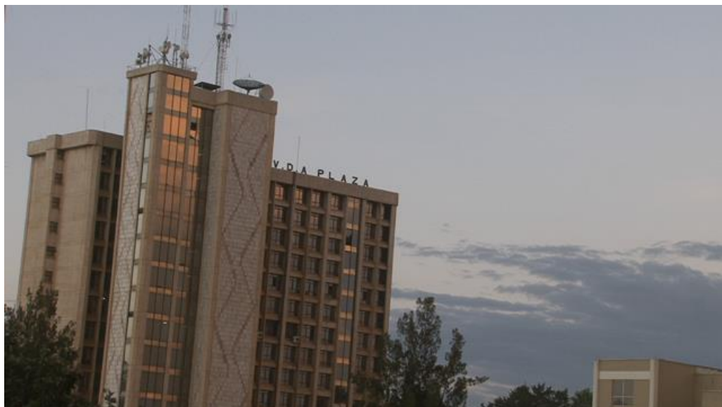
Plate 18: Kerio Valley Development Authority, constructed in late 1980's. 255 Source: https://www.kenyans.co.ke/files/styles
