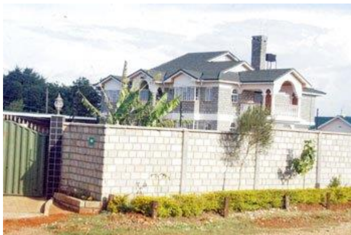
Plate 14: A Residential House in Elgon View Estate, Eldoret Source: Photo taken by researcher on 20 th July 2020
