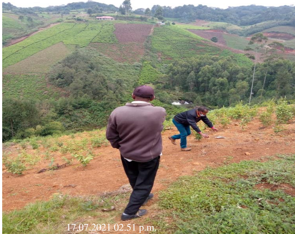
A landslide site in Kirangi Sub-Location, Mbugiti Location in Gatanga Sub-County, Murang'a County
