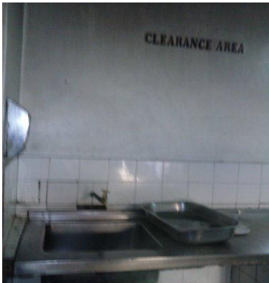
Plate 4.9: Kitchen with designated work areas
