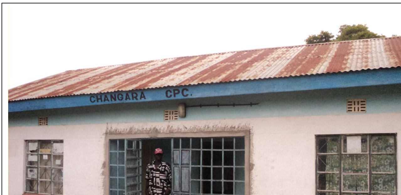
Building housing Changara community power centre under Bungoma DBSC
