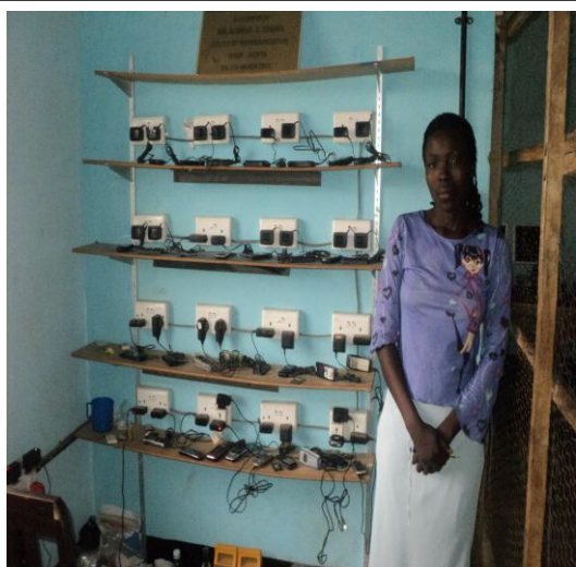
Mobile phone charging project at Changara (Bungoma DBSC)
