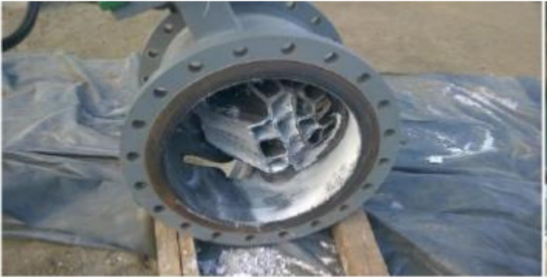
**Figure 2.4:** Steam valve with silica scales from Olkaria II power plant
