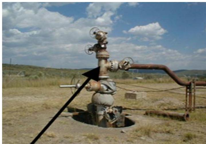
**Figure 4.11:** T-Connection on well 37B
