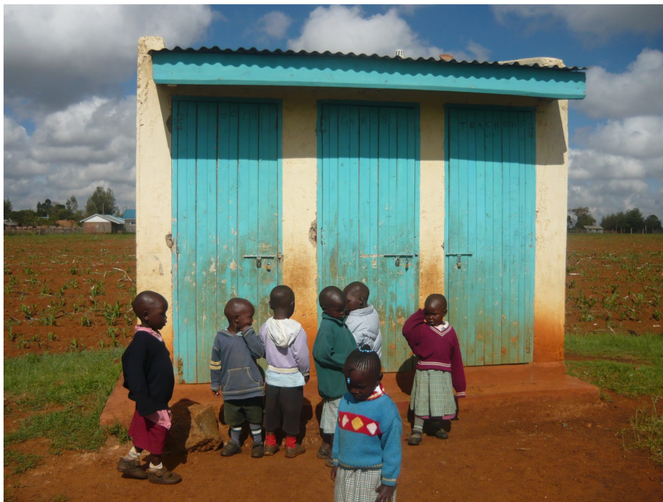
Fig. 5.4.2.4 A Toilet constructed through CSG
