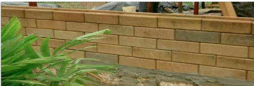
**Figure 4.3 A wall built using interlocking stabilized soil blocks**
