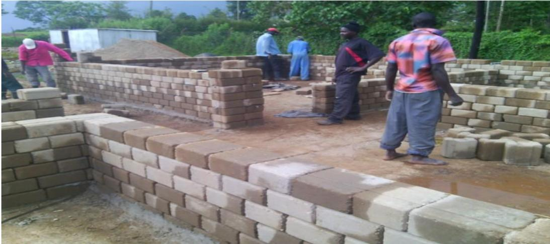
**Figure 4.2. A house under construction using ISSB**
