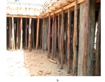
Plate 1 Two types of scaffolding commonly used in buildings. Type 1 (a) can use thin and longer poles while type 2 (b) will need thicker, shortter and stronger material.
