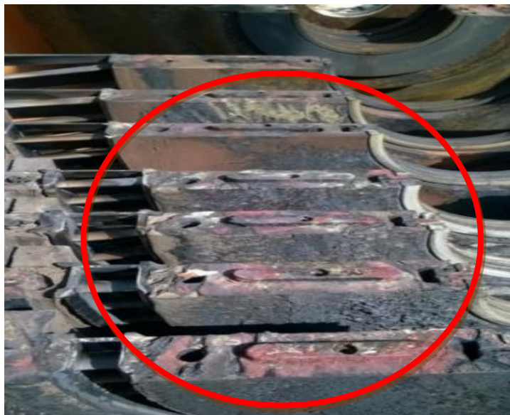
Figure 1.3: Eroded and steam gouged diaphragms (Source: Researcher, 2019)
