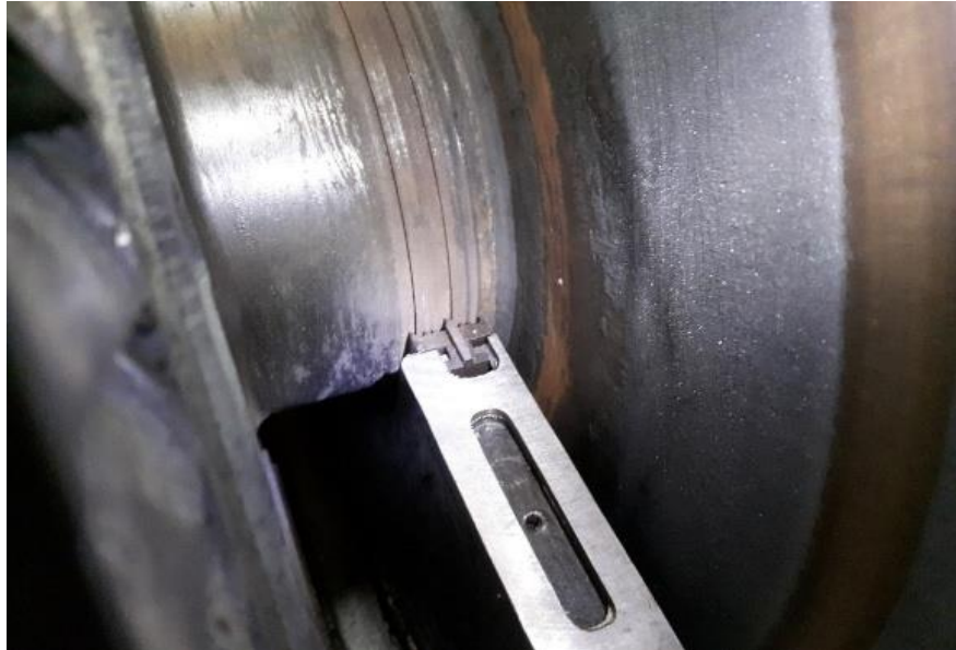
Figure 3. 11: Repaired and installed diaphragm with rotor (Source: Researcher, 2019)
