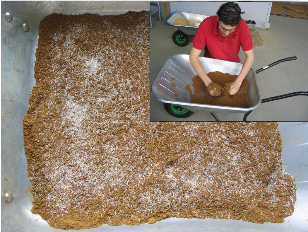
Figure 5.1 Soil-fibre manual mixing
