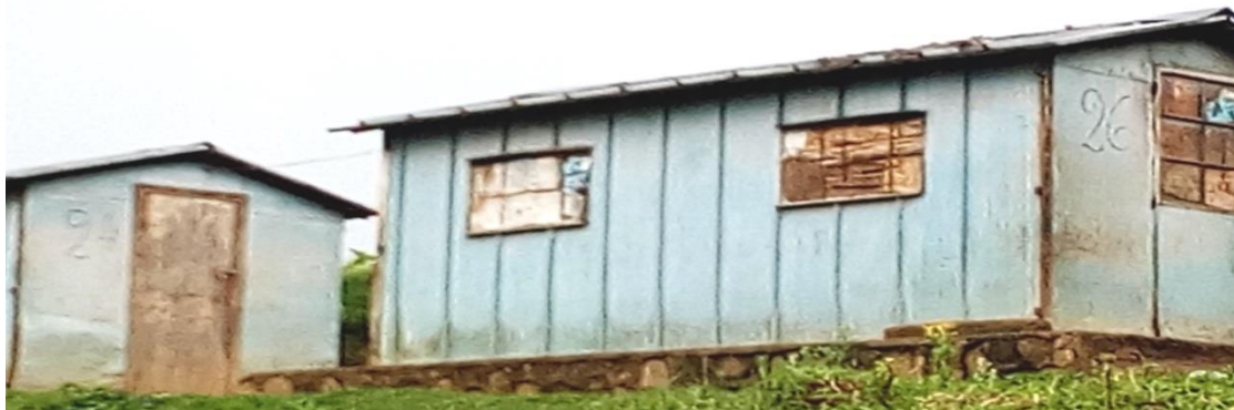
Plate 4.4. Accommodation for workers
