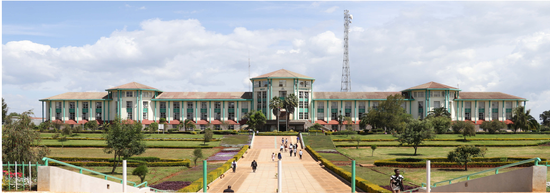
Moi University Administration Building, Main Campus
